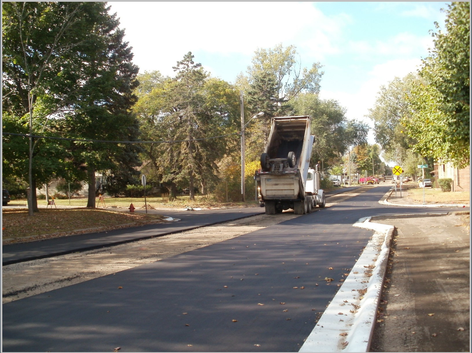
New Asphalt Installation – 1st Lift
