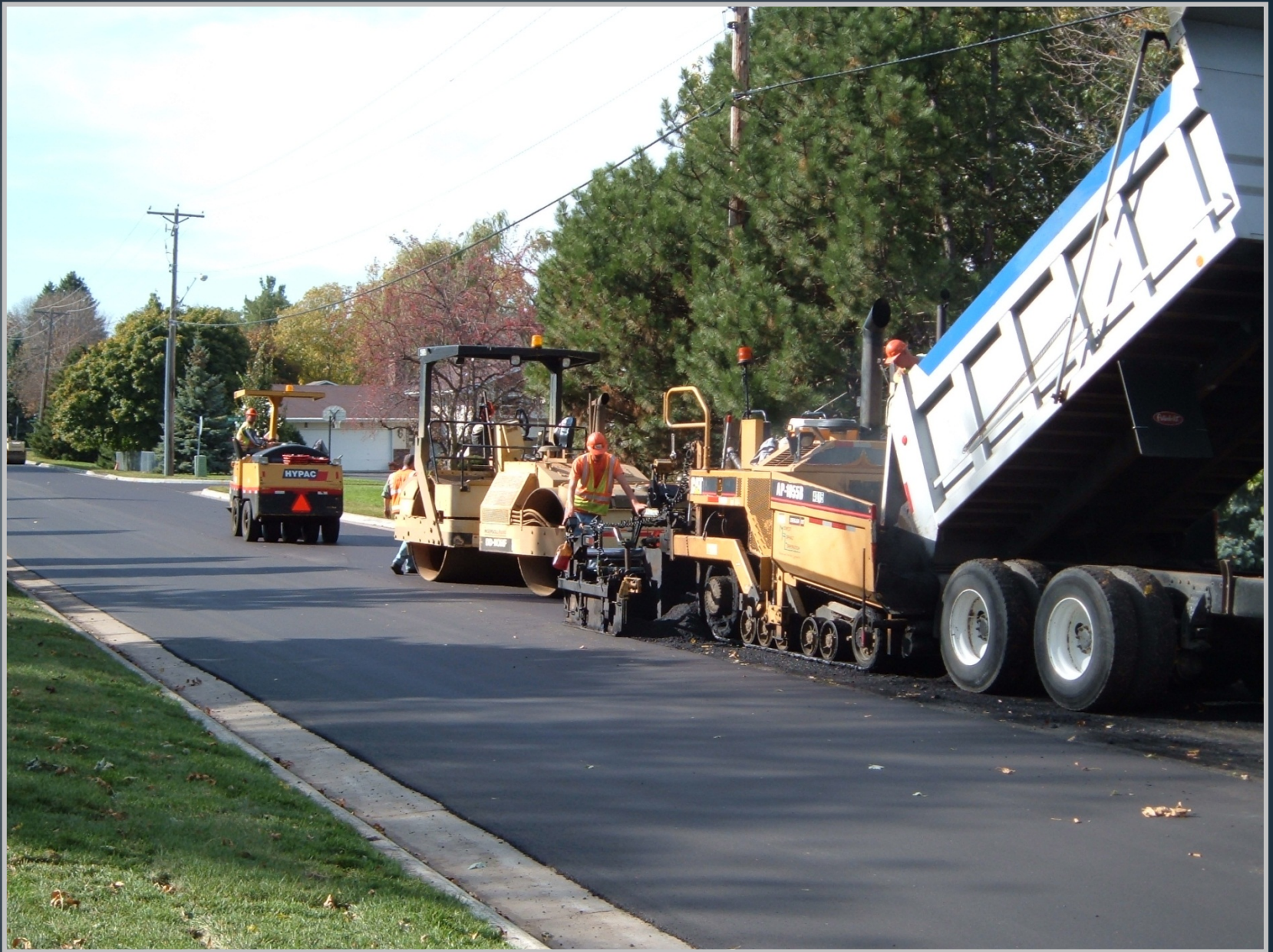
New Asphalt Installation – 2nd Lift
