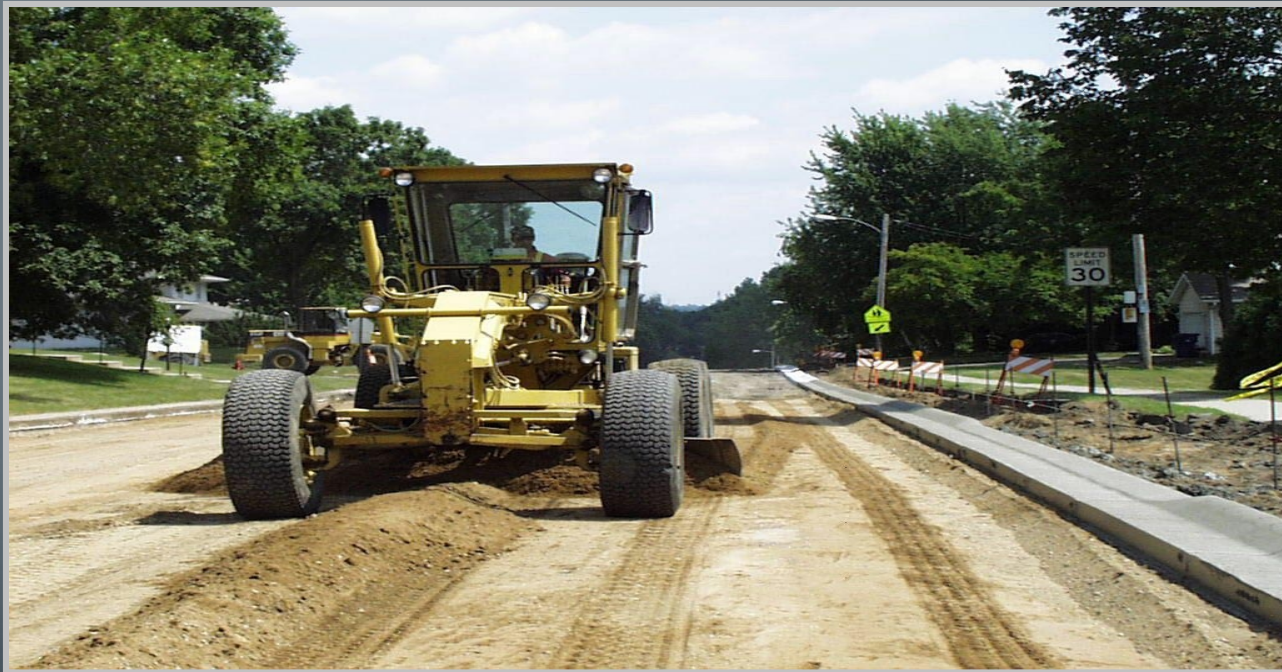
Grading Aggregate Base
