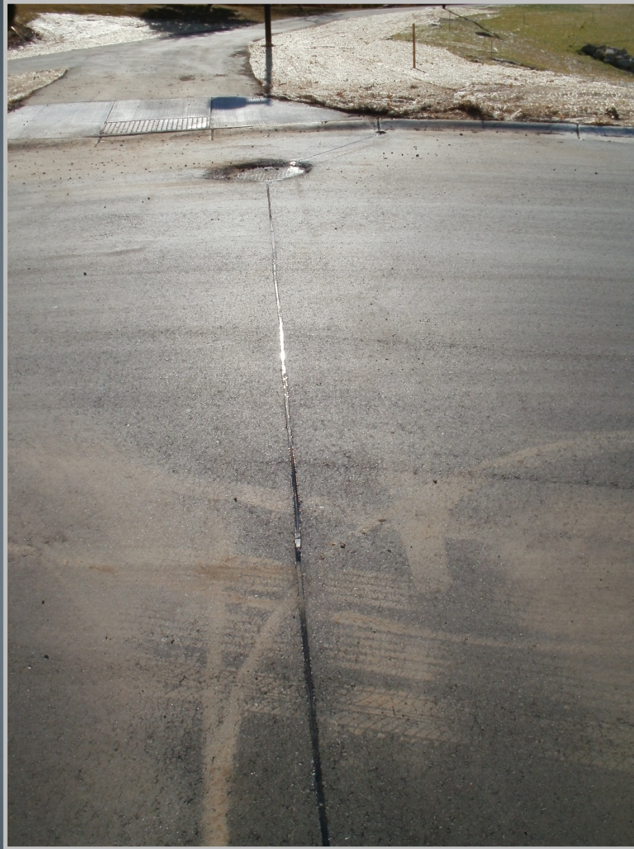
Saw & Seal Cracks
