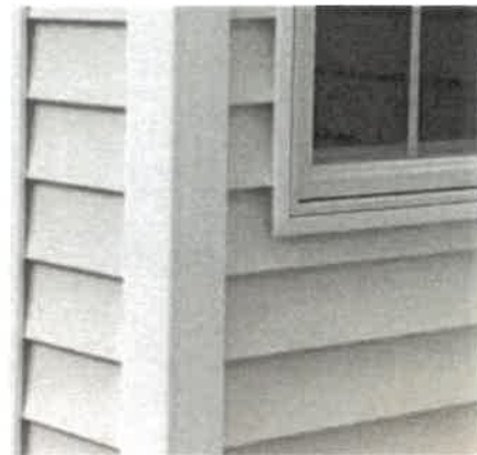
Trimworks traditional corner post.
