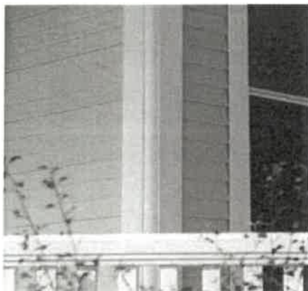
Trimworks® three-piece beaded corner post.
