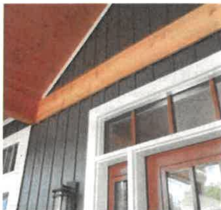
Board & Batten vertical siding accentuates gables and other areas.
