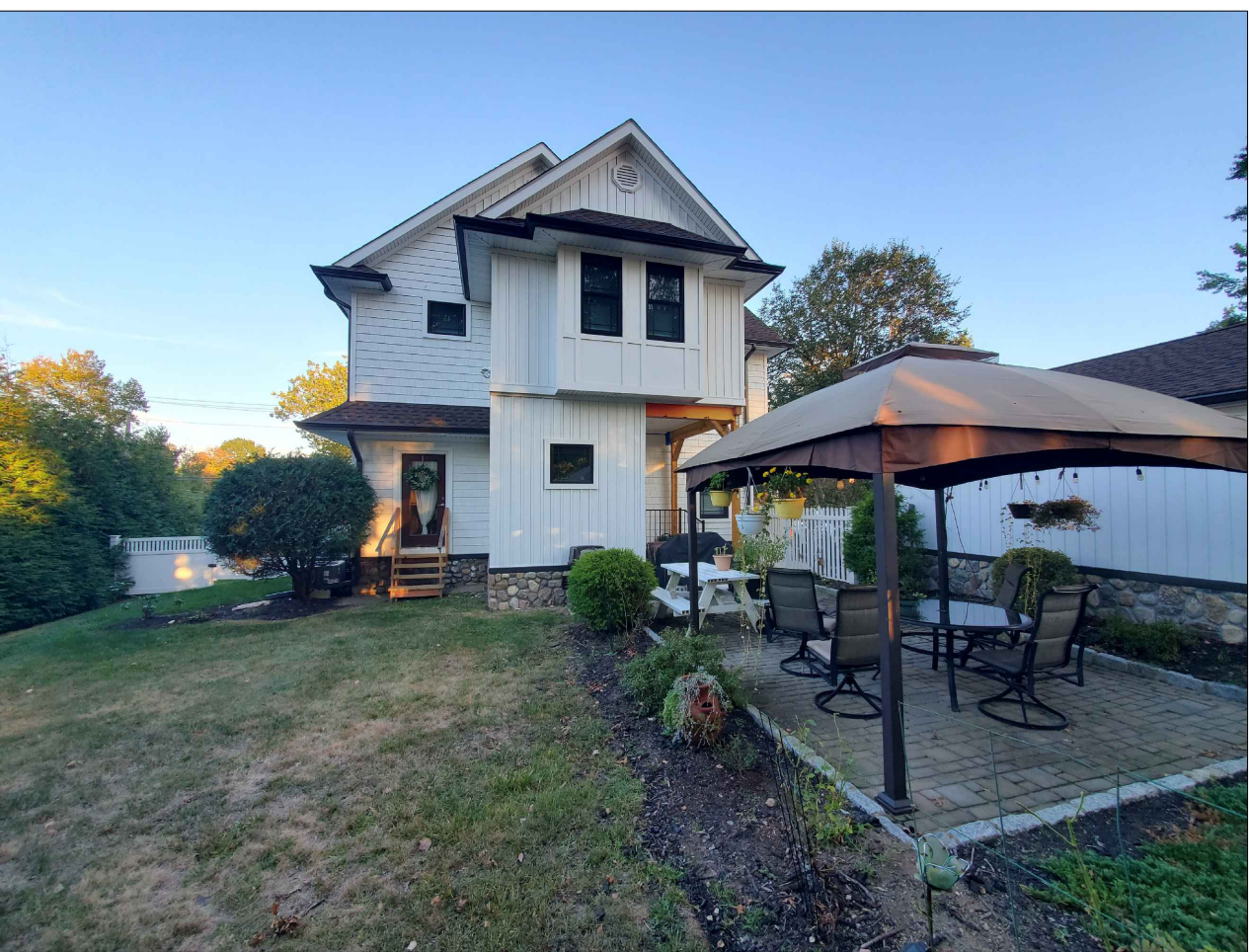
14. WEST ELEVATION @ PATIO & FUTURE DECK
