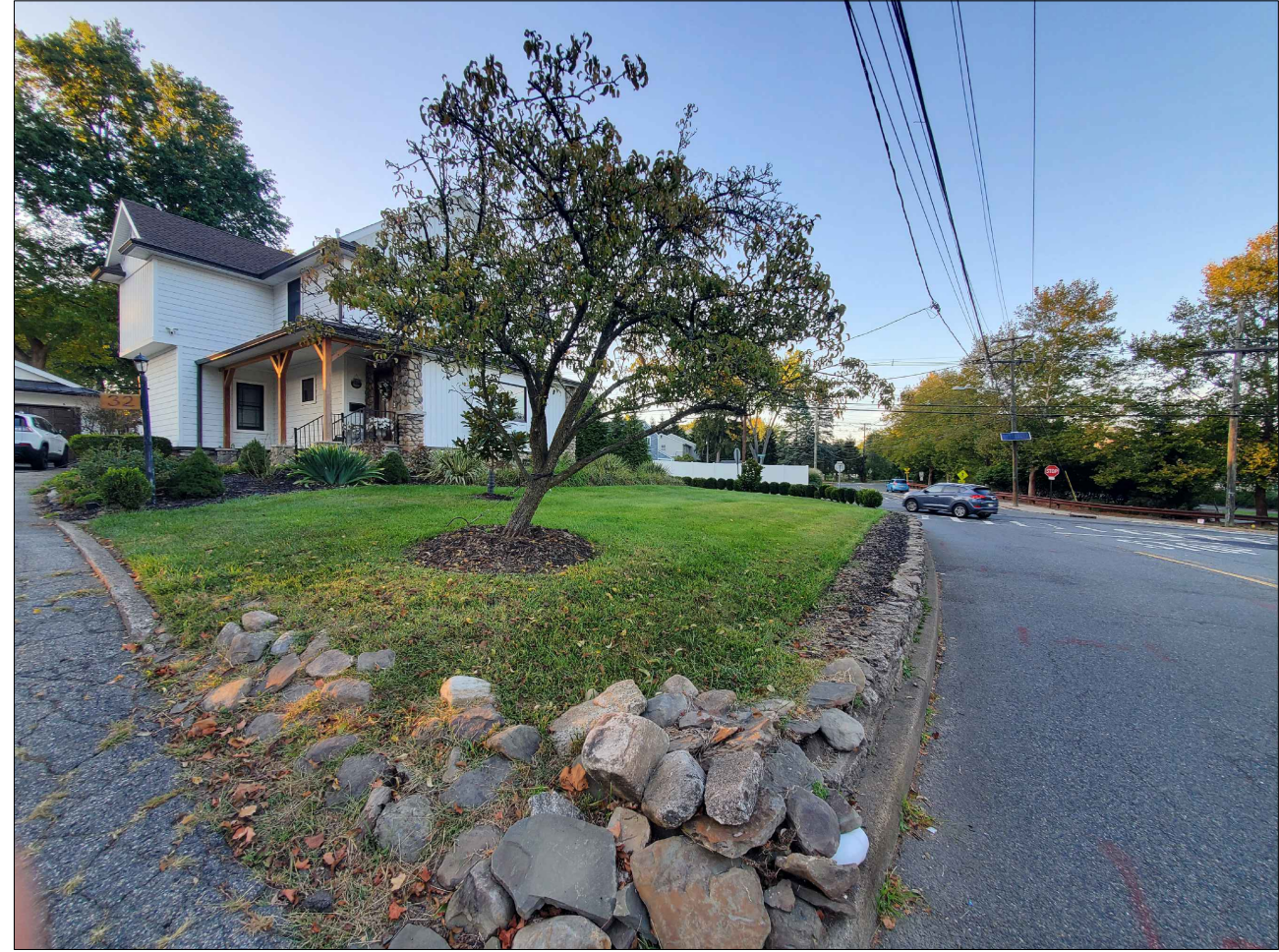
5. CURB & DRIVEWAY @ 32 HOPPER AVENUE
