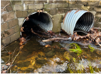
Ap Gates Outlet end of Culvert
