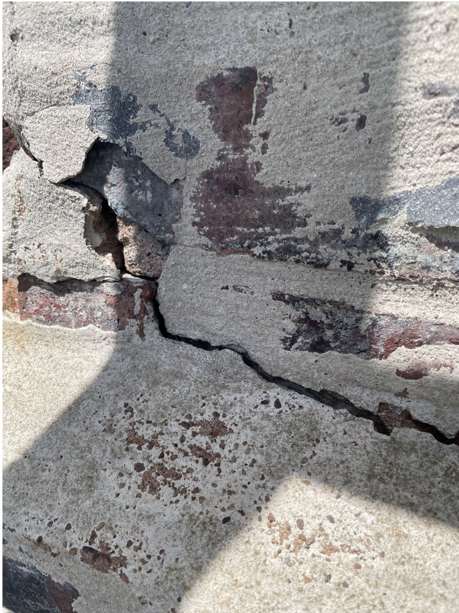
Photo 8: Additional cracks observed in exterior wall.
