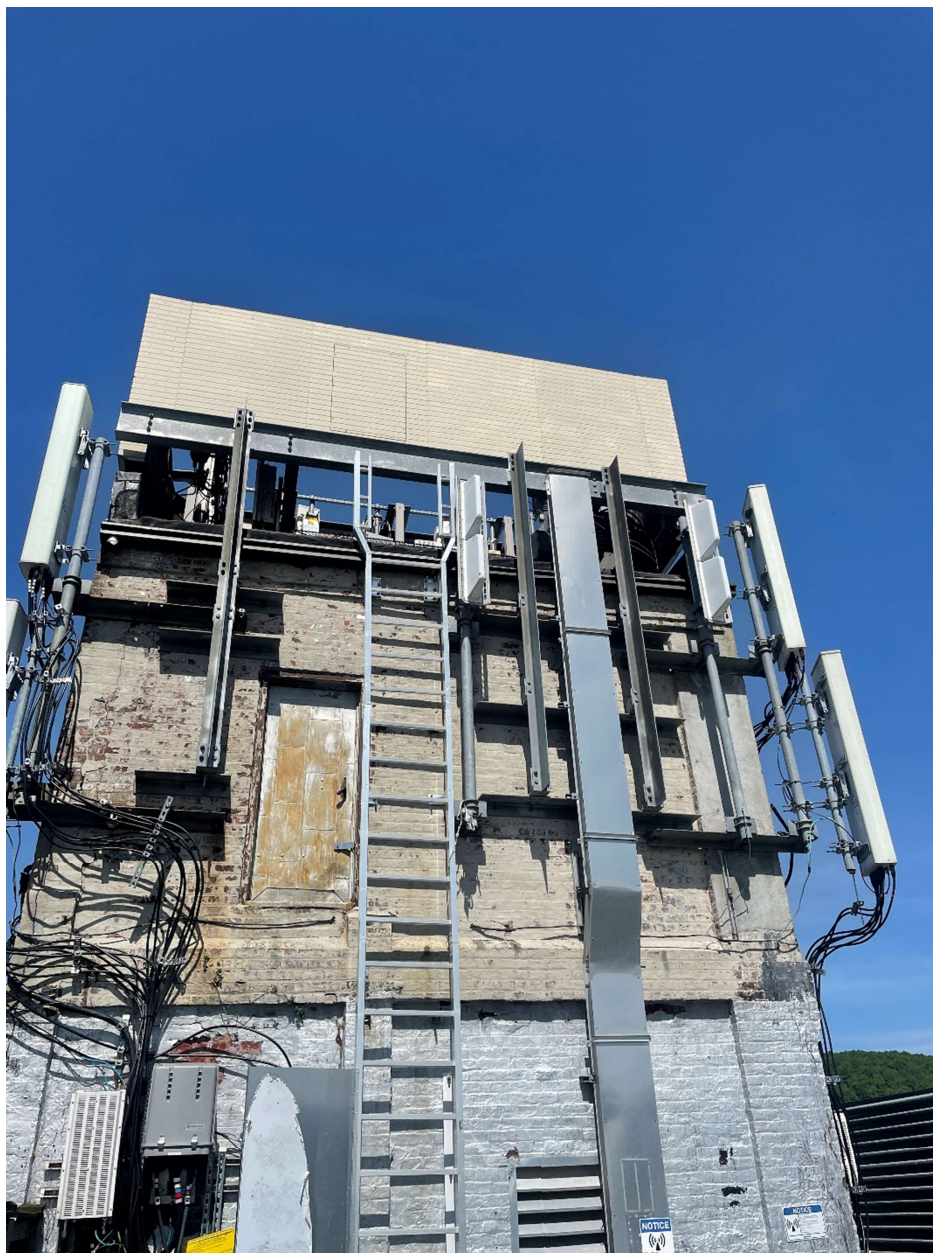
Photo 6: AT&T's coaxial run in cable tray.
