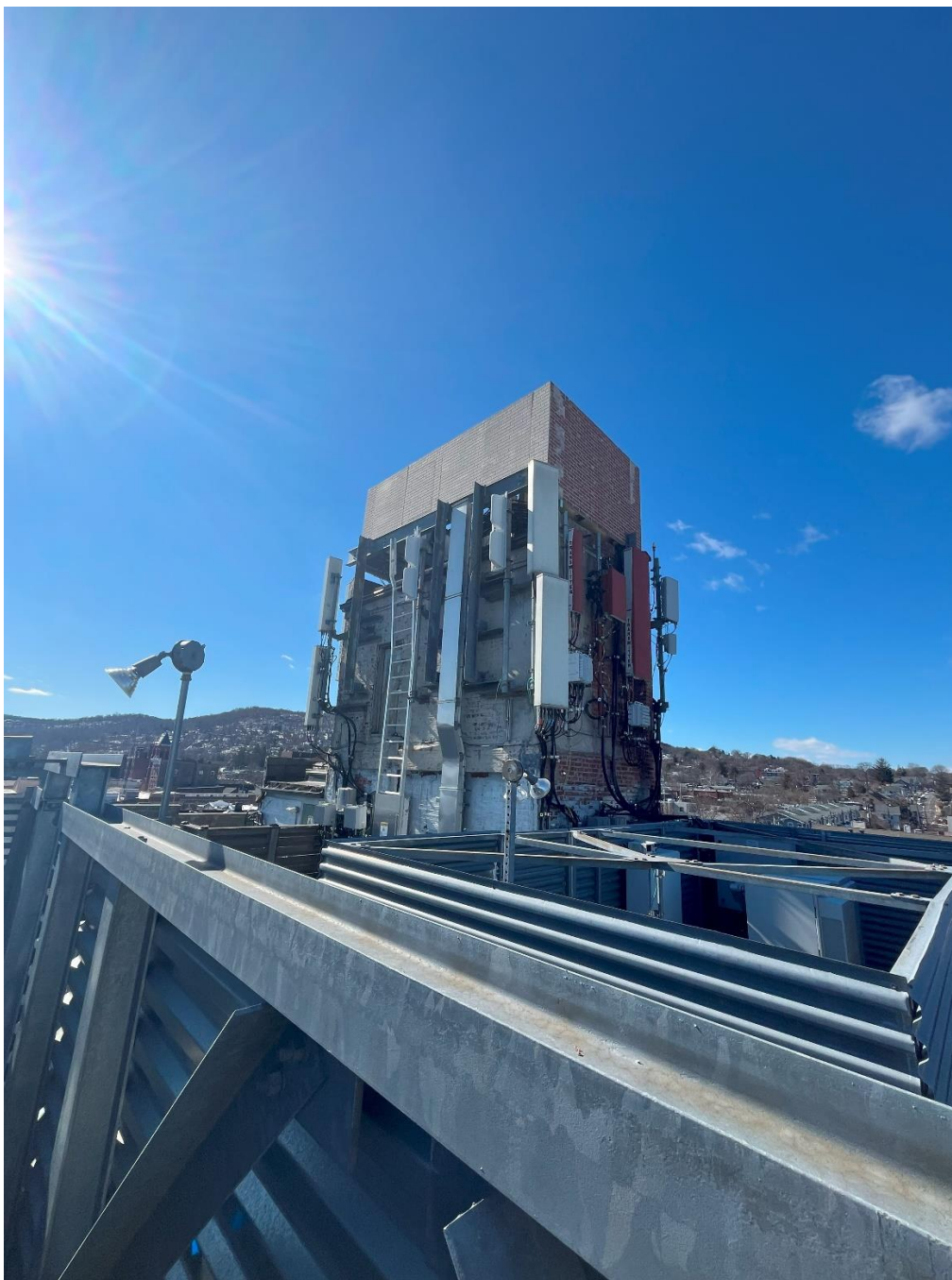
Photo 2: AT&T's Cable Tray and Alpha Sector (beyond screenwall).
