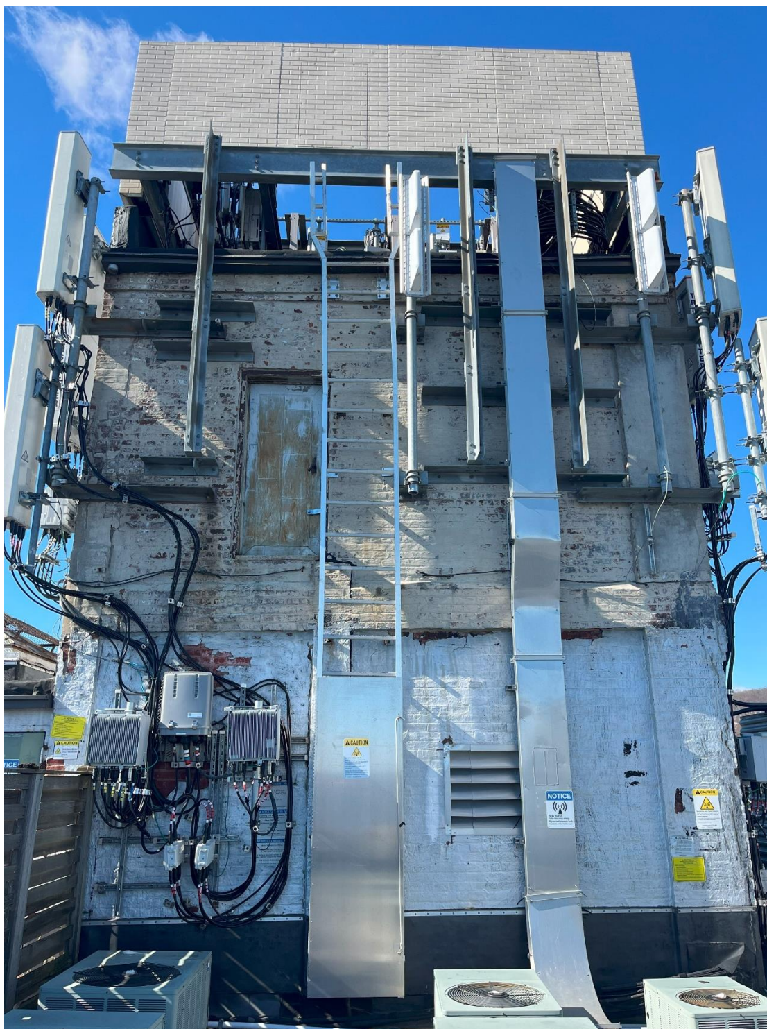
Photo 6: AT&T's coaxial run in cable tray.
