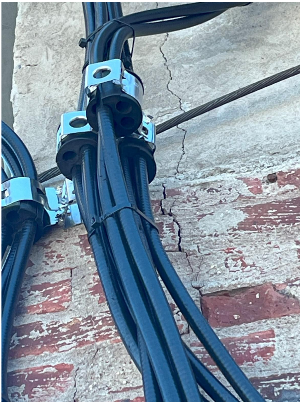
Photo 9: Additional vertical cracks observed on alpha sector bulkhead exterior wall elevated at approximately 15' at the corner SE edge of wall
