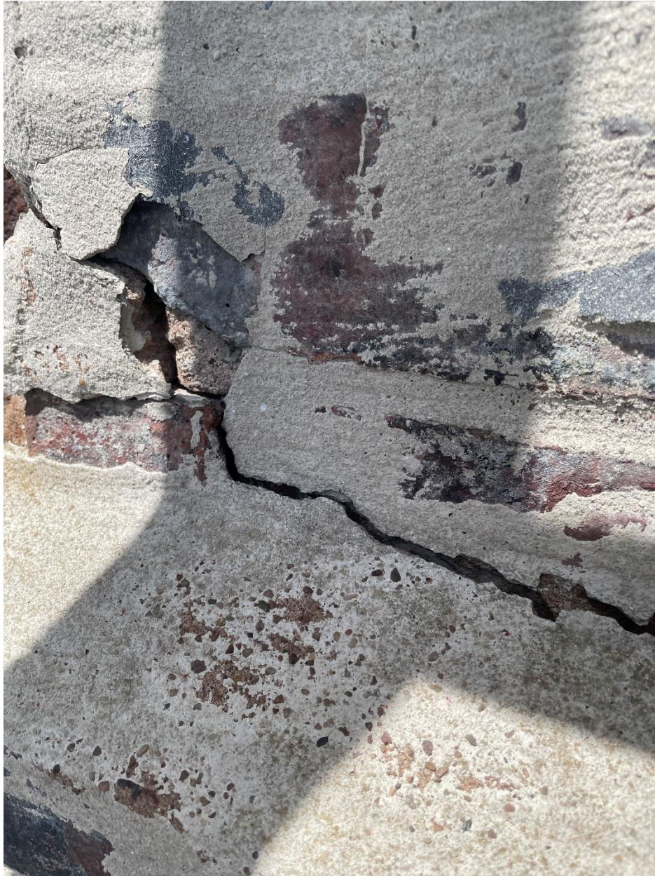
Photo 10: Additional horizontal cracks observed on the cable tray wall of the bulkhead exterior elevated at approximately 15' SE of wall mounted ladder.
