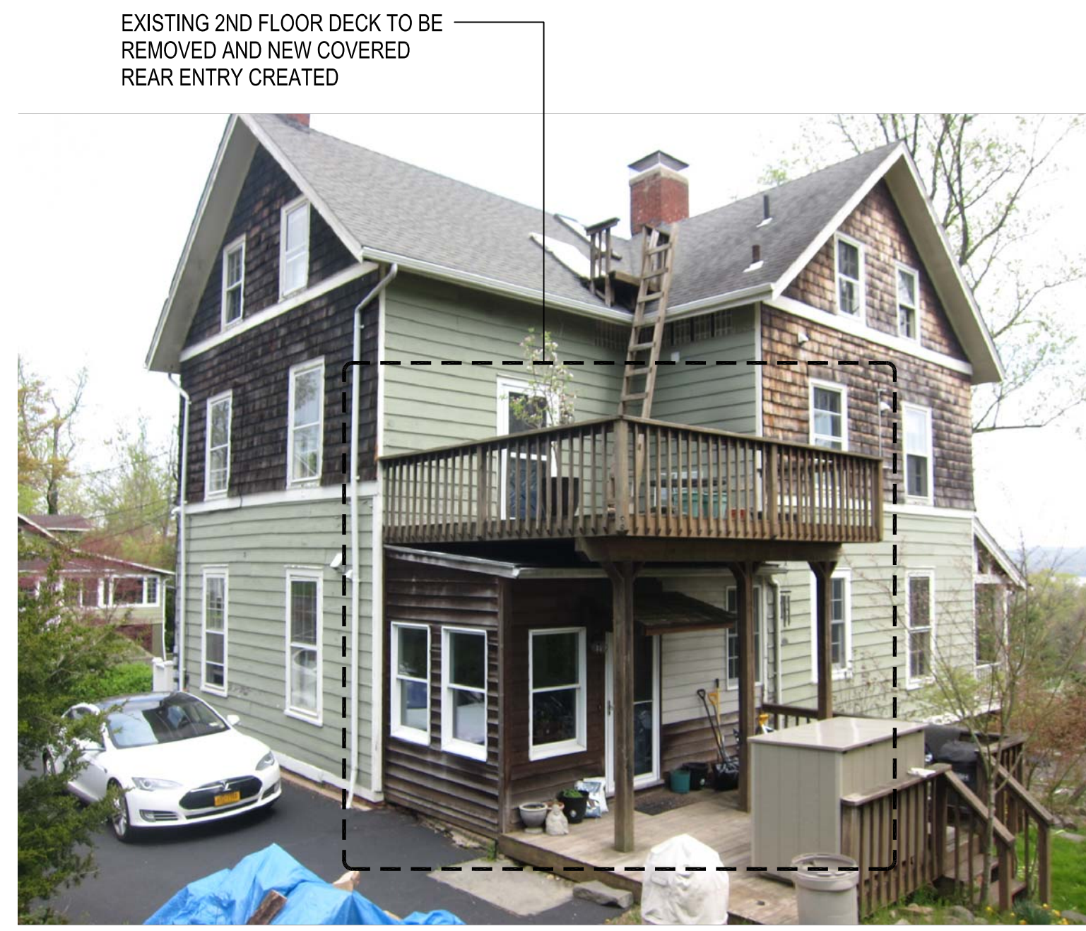
EXISTING REAR PORCH SCALE: N.T.S. SOUTH/WEST FAÇADE
