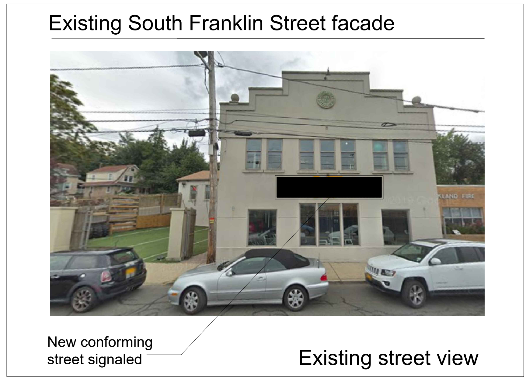
Existing South Franklin Street facade
