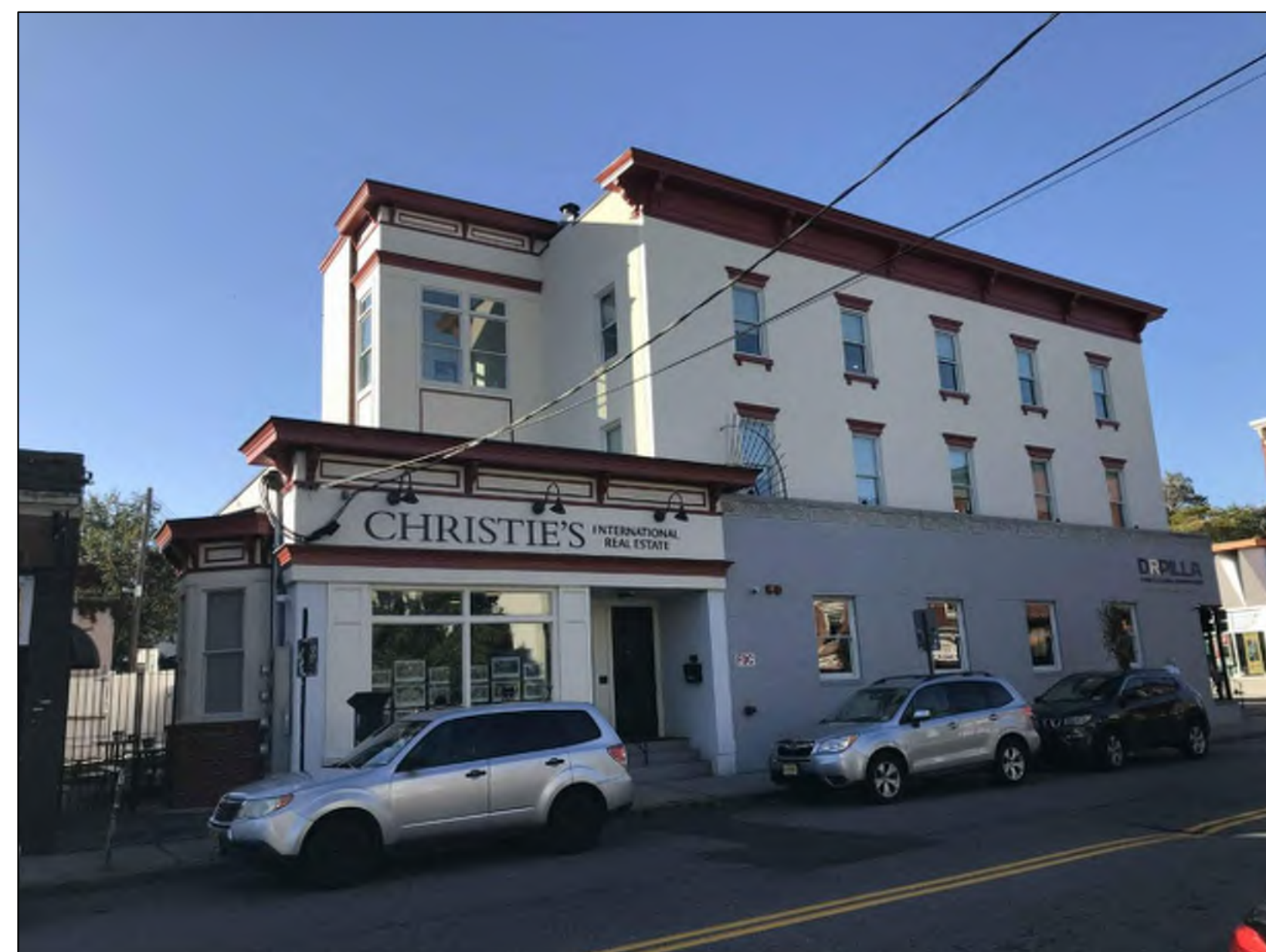
7 PHOTO 7 143 MAIN STREET - EAST ELEVATION
