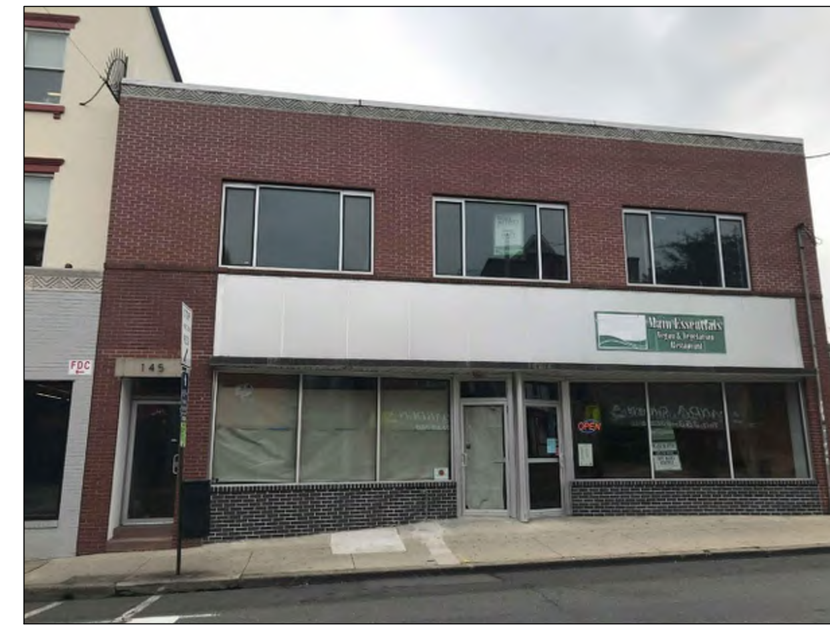
3 PHOTO 3 145 MAIN STREET - NORTH ELEVATION
