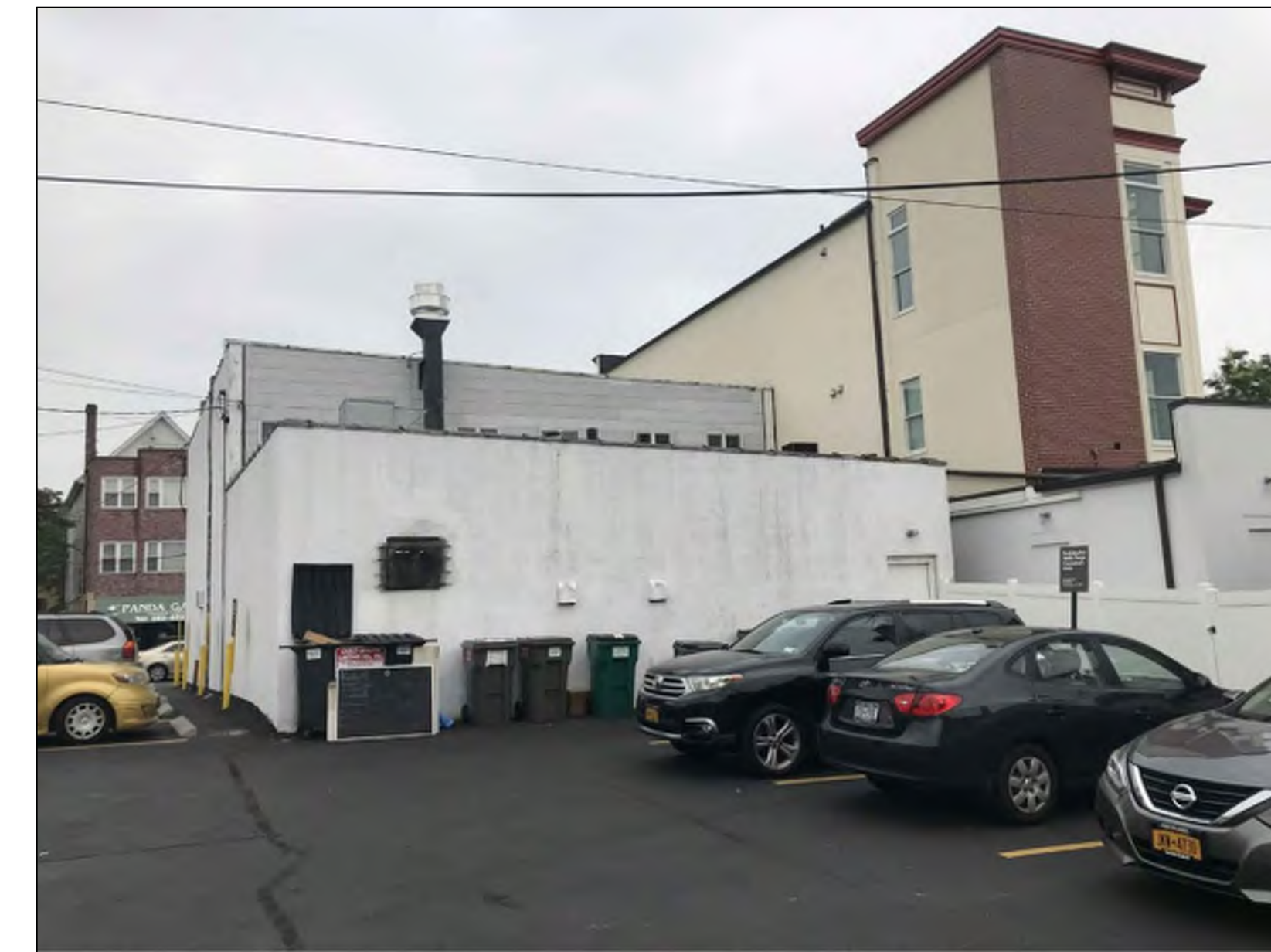
6 PHOTO 6 143 & 145 MAIN STREET - SOUTH ELEVATION
