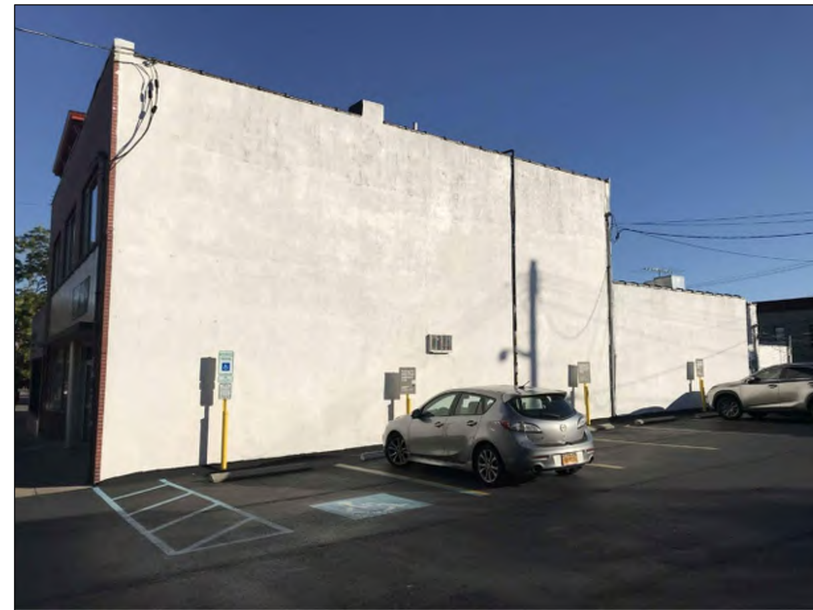
5 PHOTO 5 145 MAIN STREET - WEST ELEVATION
