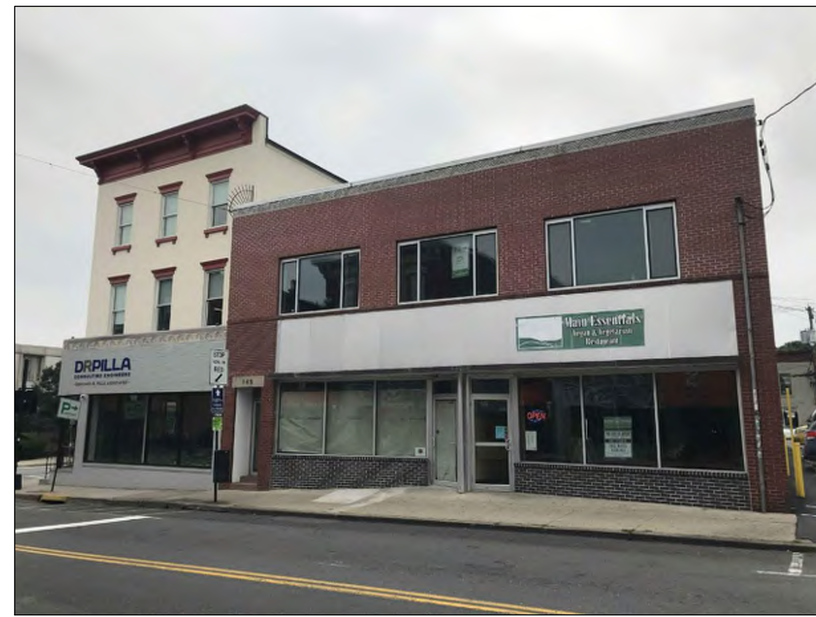
2 PHOTO 2 143 & 145 MAIN STREET - NORTH ELEVATION
