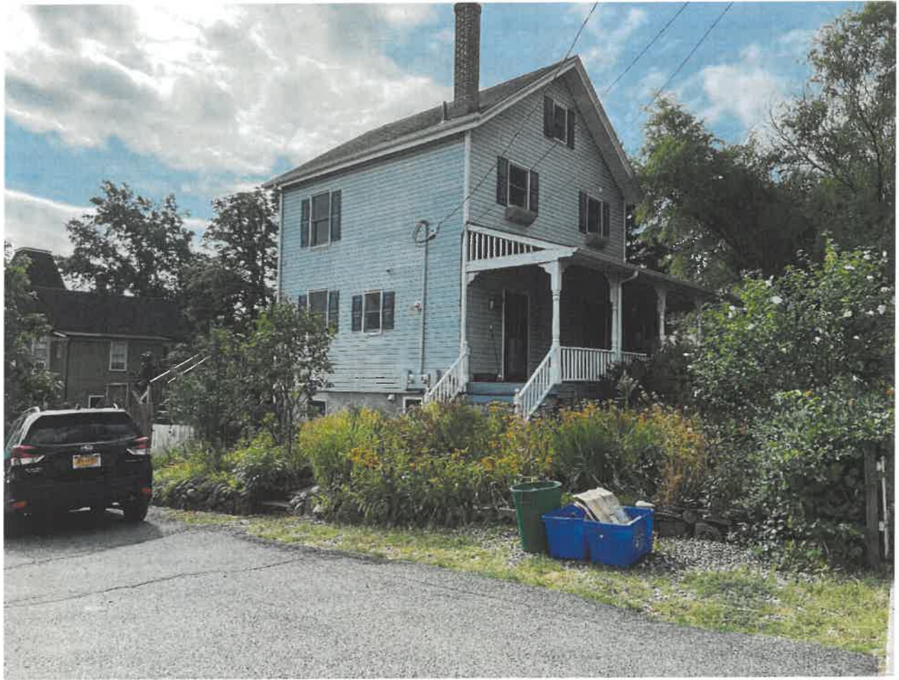
Photo 14 – 100 Cedar Hill Ave north elevation
