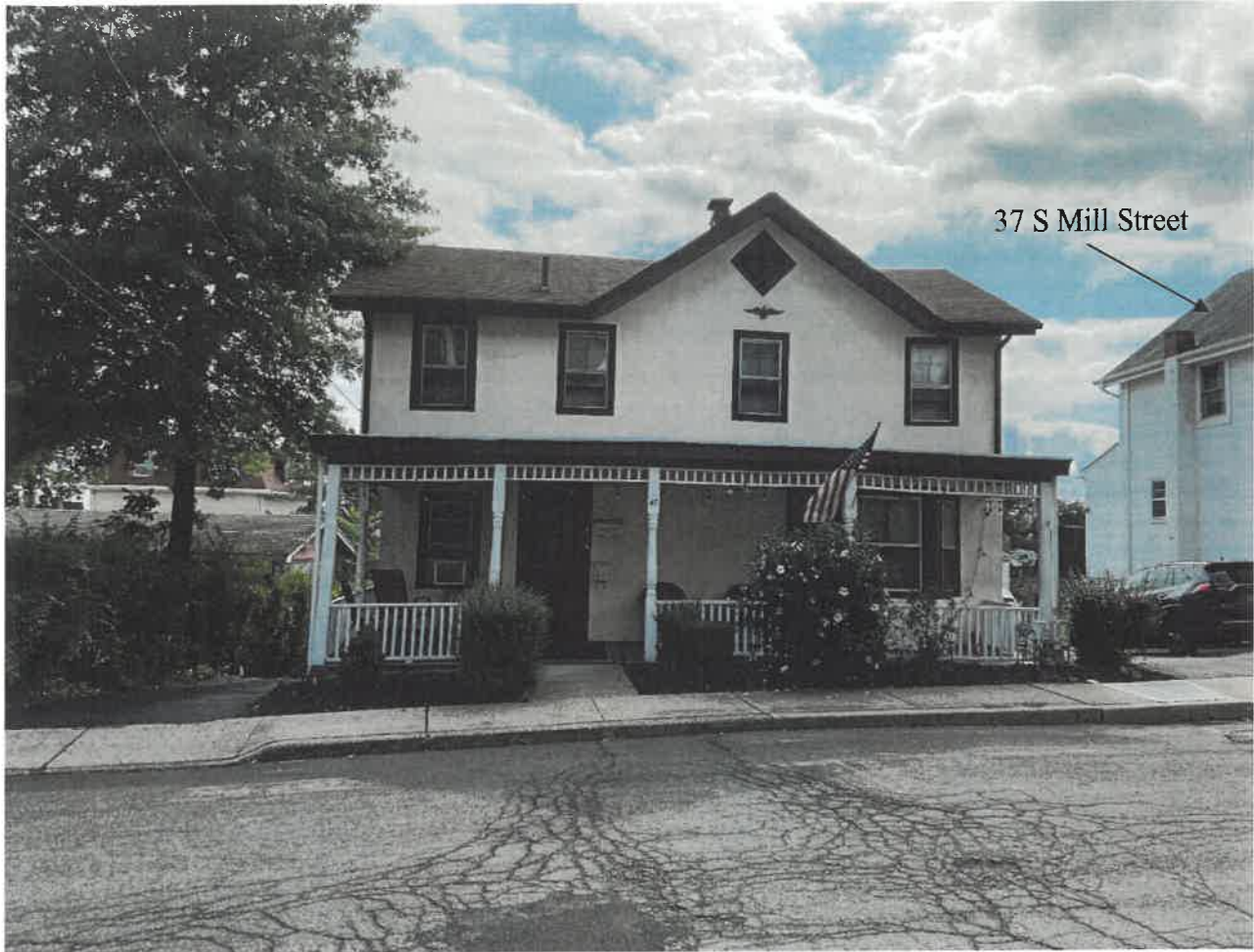
Photo 10 – 47 S Mill Street west elevation
