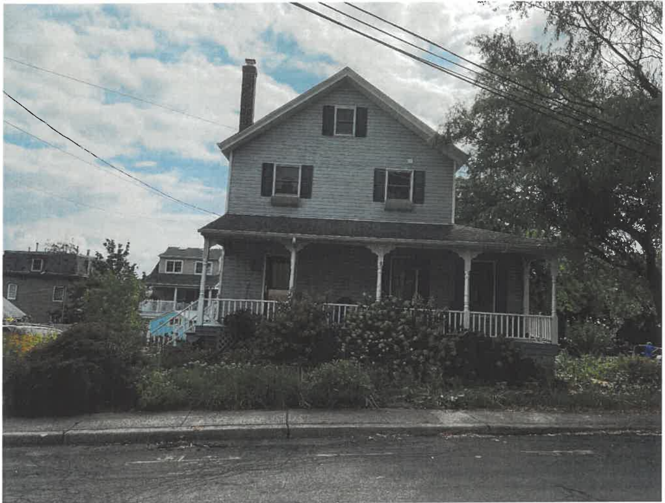
Photo 12 – 100 Cedar Hill Road west elevation
