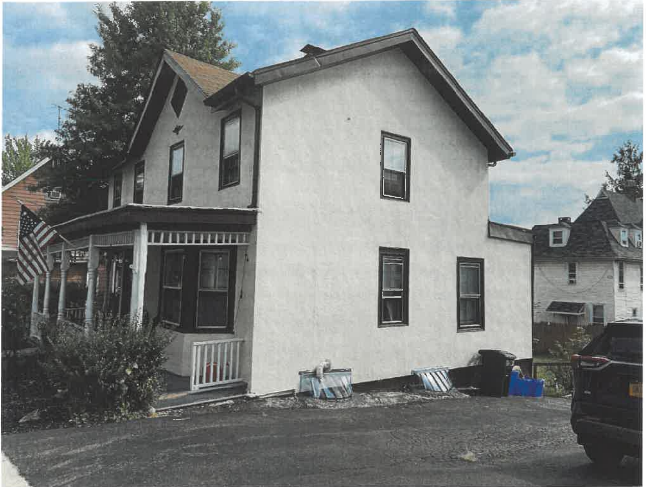
Photo 11 – 47 S Mill Street south elevation
