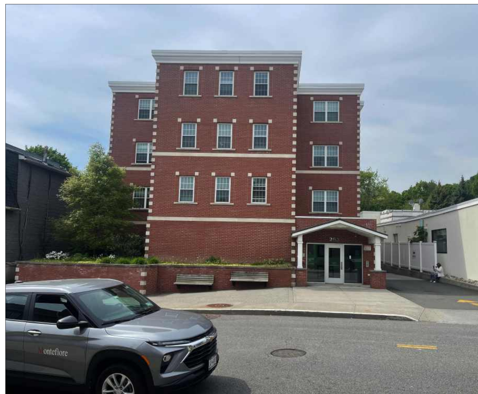
A ADJ STRUCTURE EAST (FRONT) MAIN STREET
