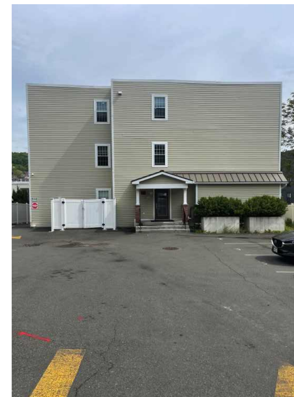
C ADJ STRUCTURE EAST (REAR) DEPEW AVENUE
