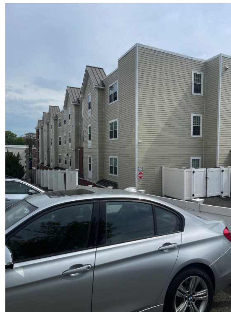
B ADJ STRUCTURE EAST (SIDE) DEPEW AVENUE
