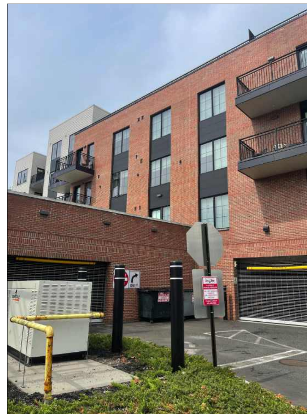
B ADJ STRUCTURE WEST (SIDE) MAIN STREET
