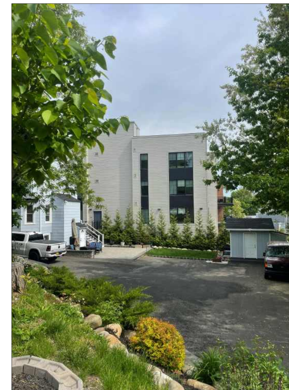
C ADJ STRUCTURE WEST (REAR) DEPEW AVENUE
