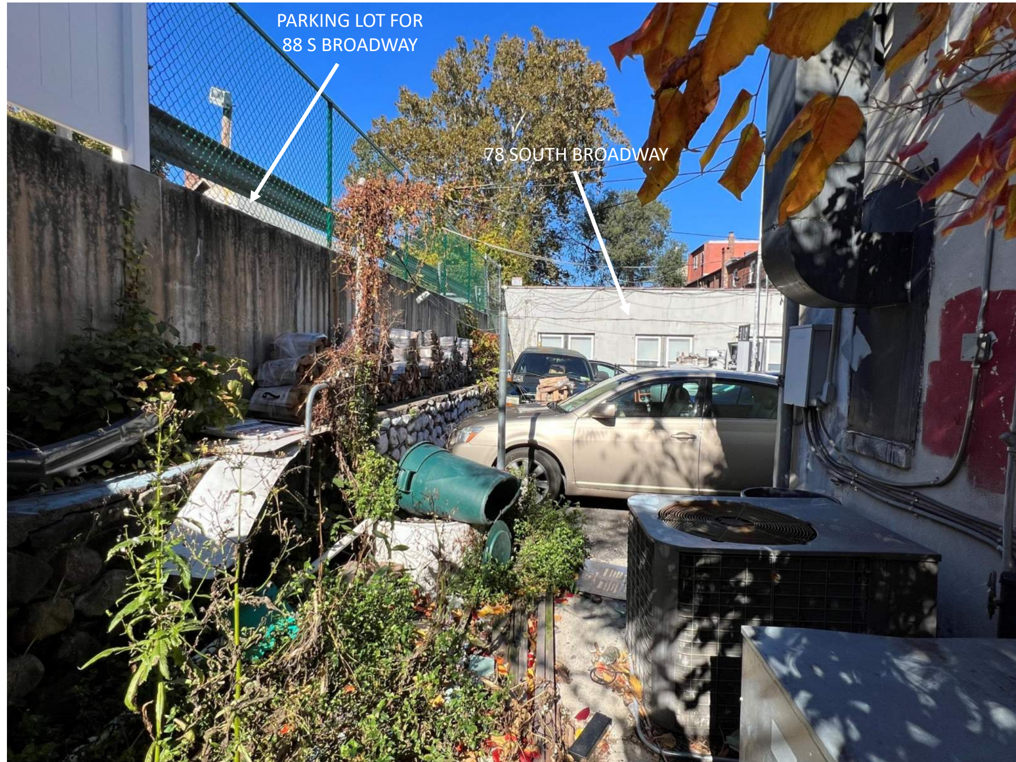
RETAINING WALL ALONG THE BACK SIDE OF 80 SOUTH BROADWAY LOOKING NORTH
