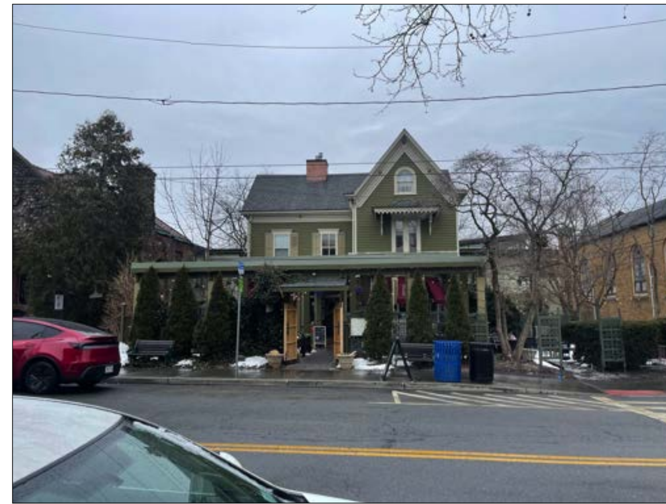
B ADJ STRUCTURE (NORTH)
