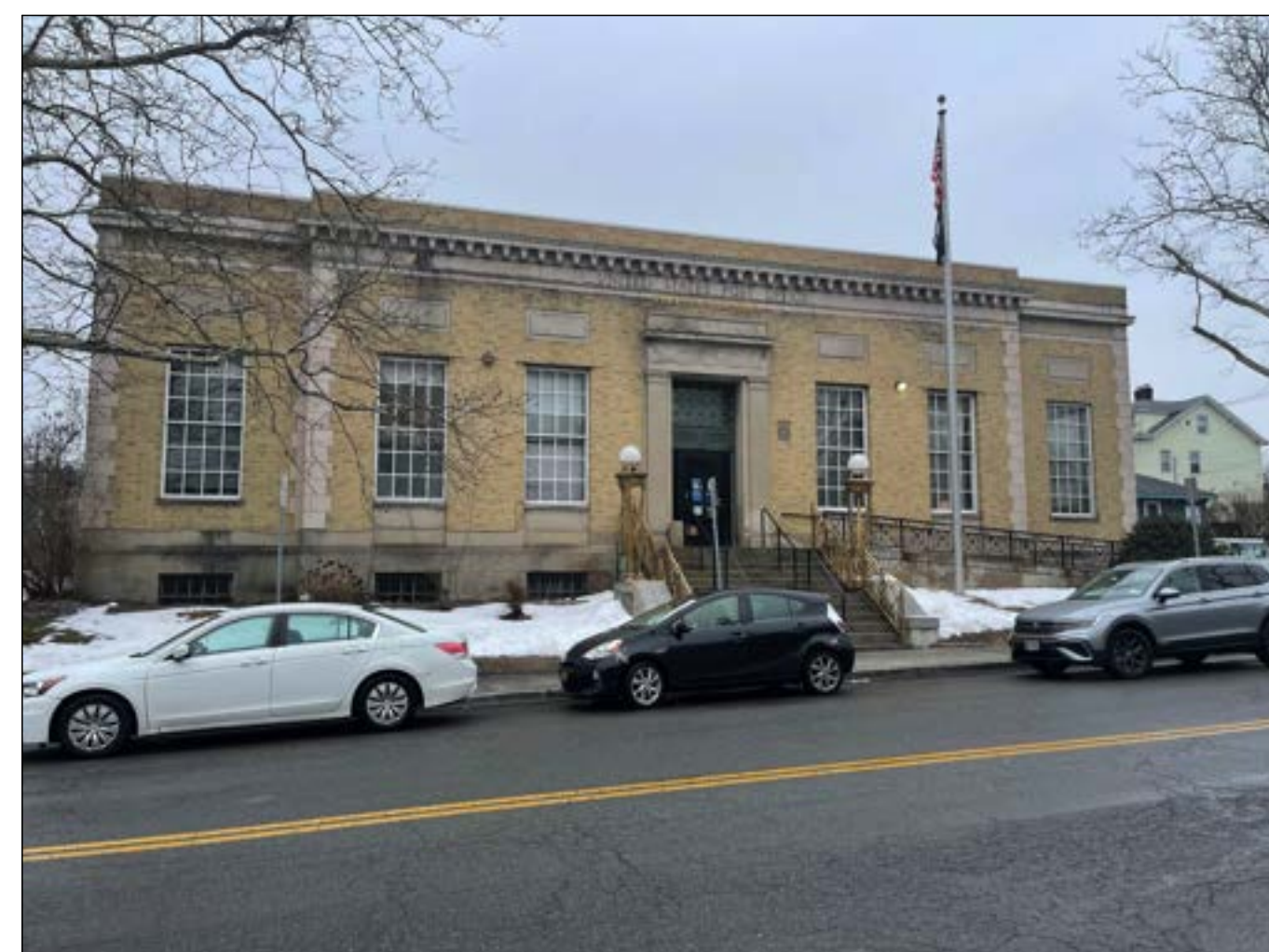
E OPP STRUCTURE (WEST)
