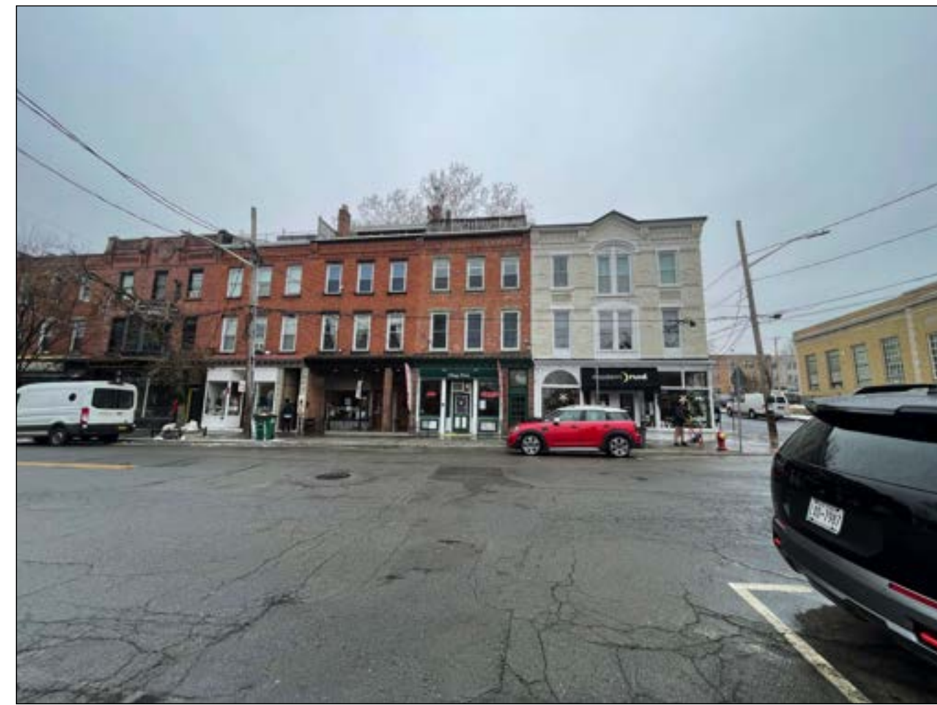
C OPP STRUCTURE (WEST)
