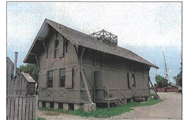
DECORATIVE TRIMWORK AROUND WINDOWS
