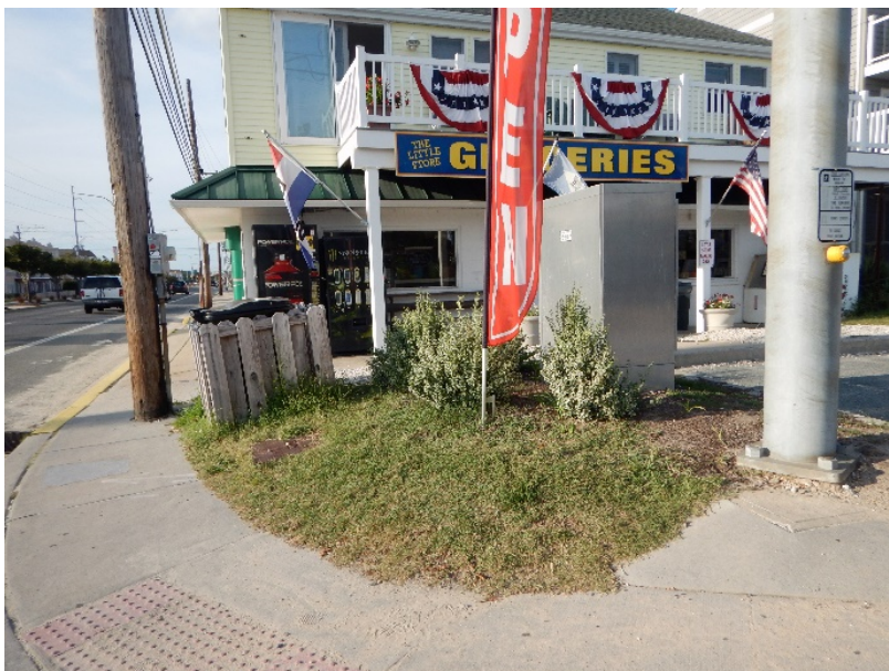
Figure 2. Existing grass island at this corner that will be converted to a bioretention facility. Gravel walkway between the island and the store will become an infiltration trench with permeable pavers.
