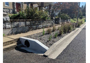
Town Hall Bioretention, Berterton, MD
