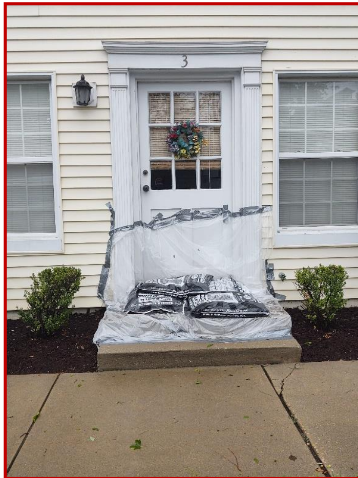
House with plastic taped over the door and sandbags to prevent flood waters from entering the house – July 2020
