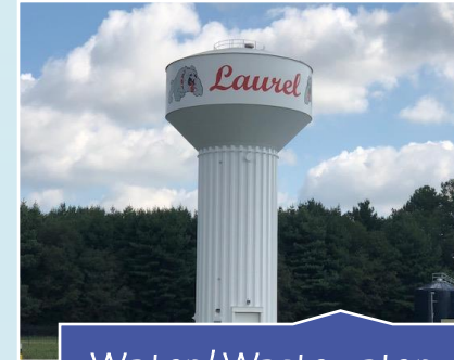
Water / Wastewater Engineering
