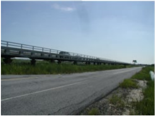
RAISED & REROUTED ROADWAYS
