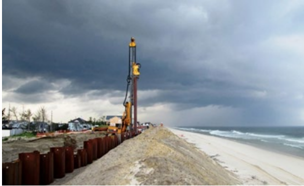
BURIED FLOODWALL / STRUCTURAL DUNE
