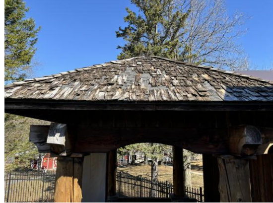
Zoo Visitor's Center – Cedar Shingles deteriorated and falling off.
