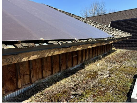
Zoo Visitor's Center – Sloped Cedar Shingle Roof currently tarped.
