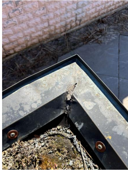
Zoo Visitor's Center – Living Roof System scupper, gravel stop, and sealant deterioration.
