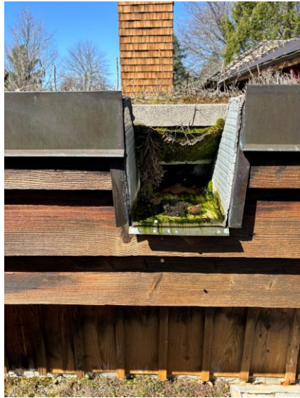
Zoo Visitor's Center – Living Roof System scupper, gravel stop, and sealant deterioration.
