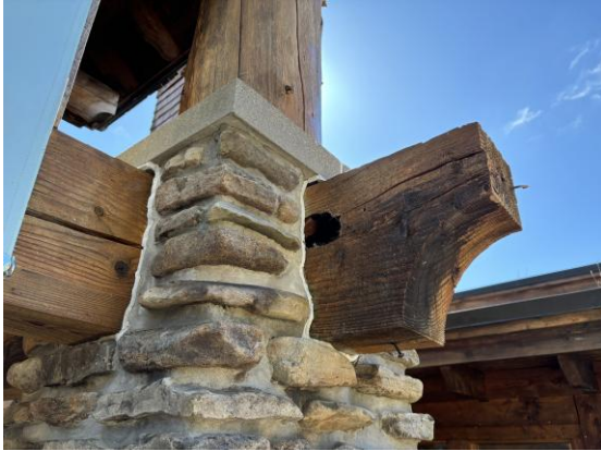
Zoo Visitor's Center – Timber frame and sealant deterioration.
