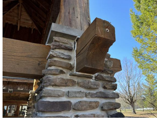
Zoo Visitor's Center – Timber frame and sealant deterioration.
