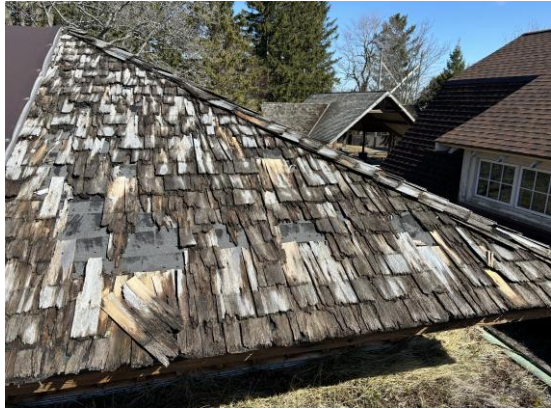
Zoo Visitor's Center – Cedar Shingles deteriorated and falling off.
