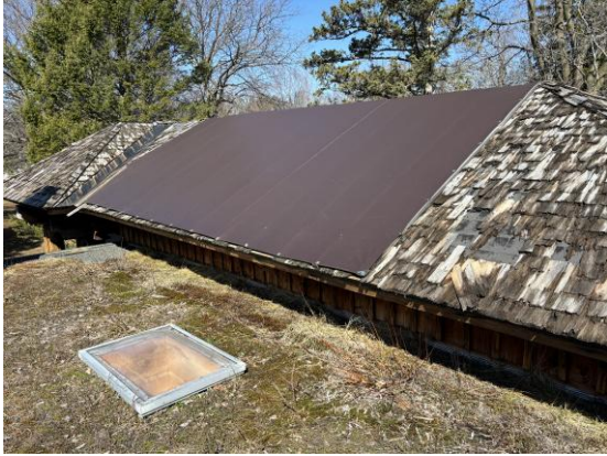
Zoo Visitor's Center – Sloped Cedar Shingle Roof currently tarped.
