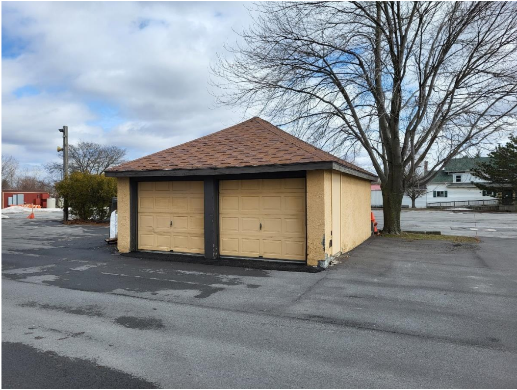
Above: A view of the existing garage on the subject parcel.
