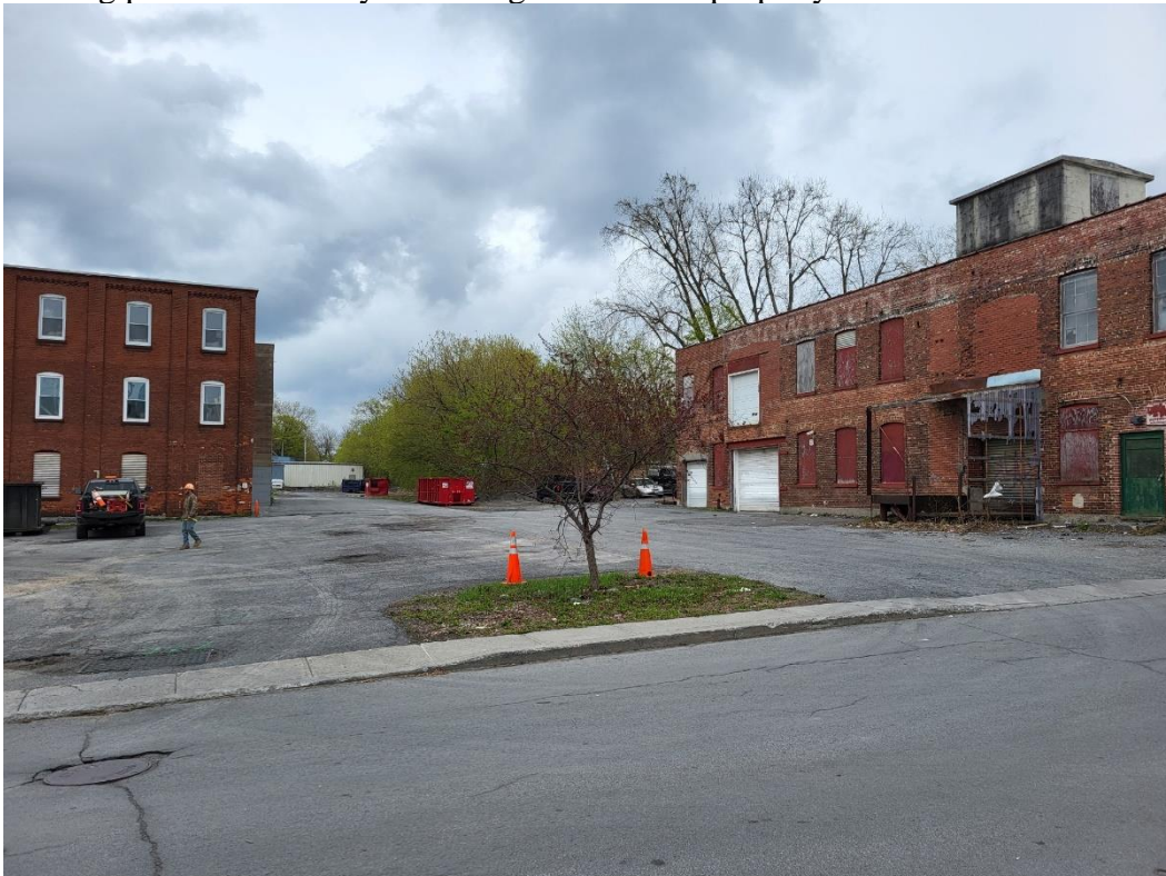
Below: A view looking east across Polk Street of the existing surface parking area at 176 Polk Street, with the existing pavement already extending to the south property line with 154 Polk Street.
