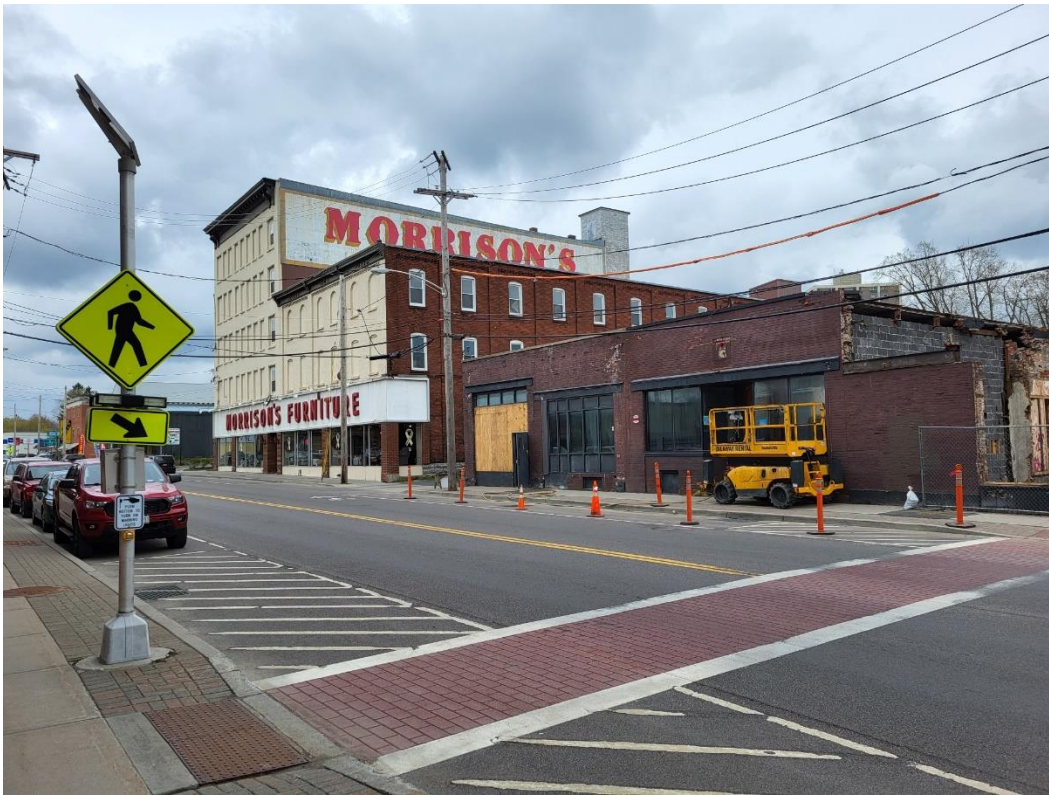
Above: A view of the existing Rectangular Rapid Flash Beacon (RRFB) and enhanced crosswalk across Factory Street with brick pavers. The RRFB on the south side does not appear in these photos as it was temporarily removed during demolition.
