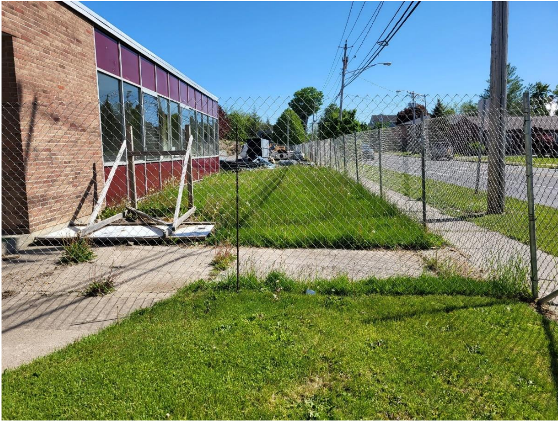
Above: A view looking south from the corner of Clinton and Mullin Streets of an existing lawn area along the western edge of the site (east side of Sherman Street). The one-story building proposed for demolition is at the left in the photo.
