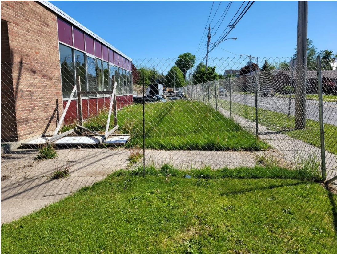
Above: A view looking south from the corner of Clinton and Mullin Streets of an existing lawn area along the western edge of the site (east side of Sherman Street). The one-story building proposed for demolition is at the left in the photo.
