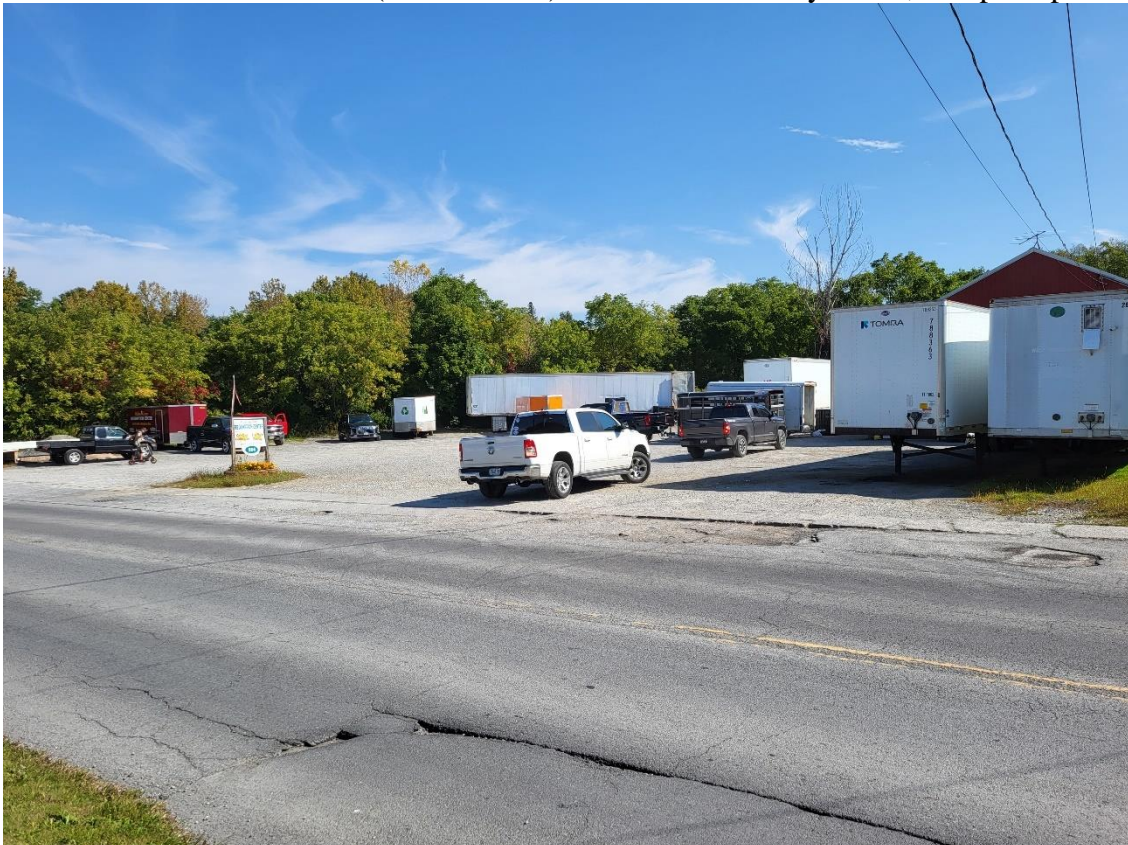
Below: A view of the south (70-foot wide) curb cut from Leray Street, as a pickup truck enters the site.
