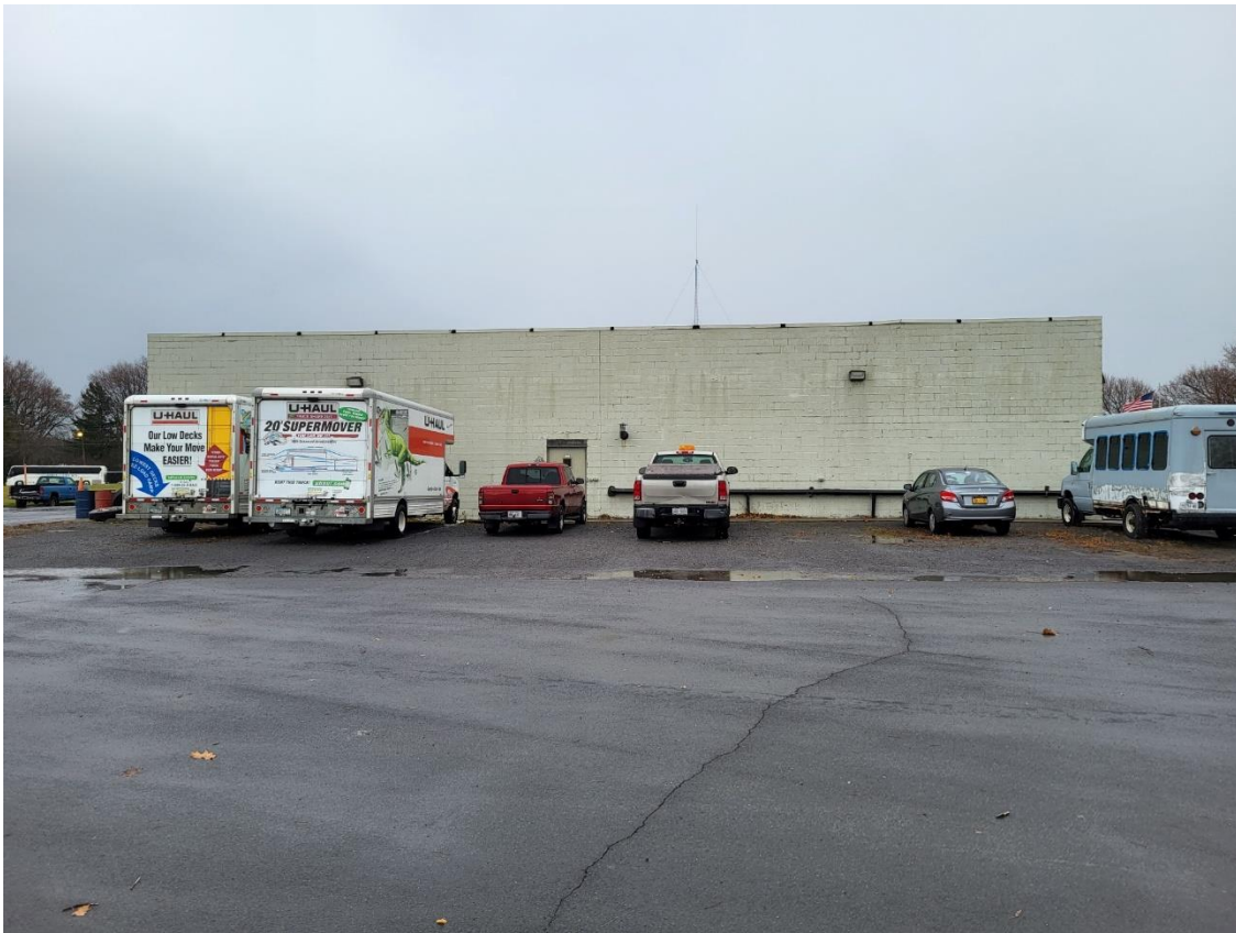
Above: A view of the existing western façade of the Hale’s bus garage building (looking east) The proposed building addition would bring the façade 50 feet closer to the camera.
