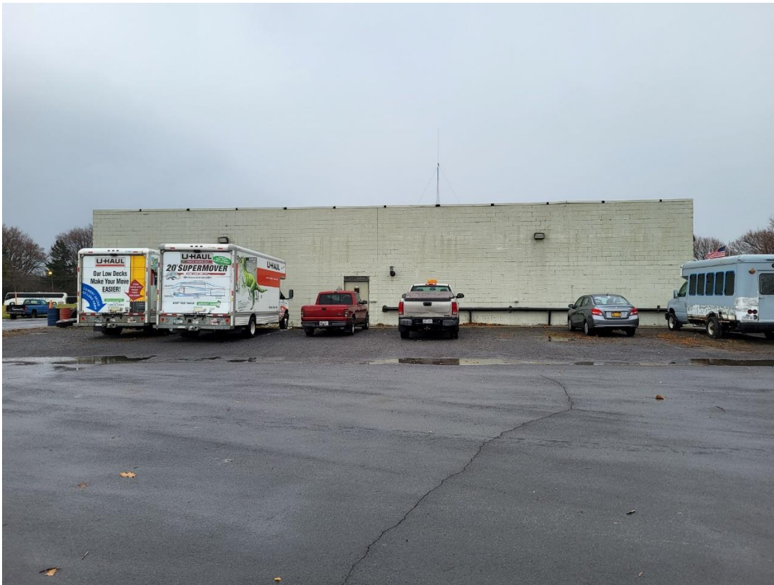
Above: A view of the existing western façade of the Hale’s bus garage building (looking east) The proposed building addition would bring the façade 50 feet closer to the camera.
