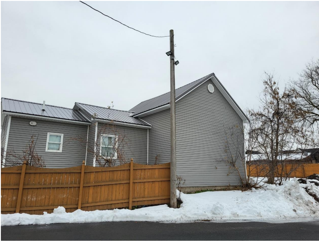
Above: The mounted light on a pole at the southern edge of the site.
