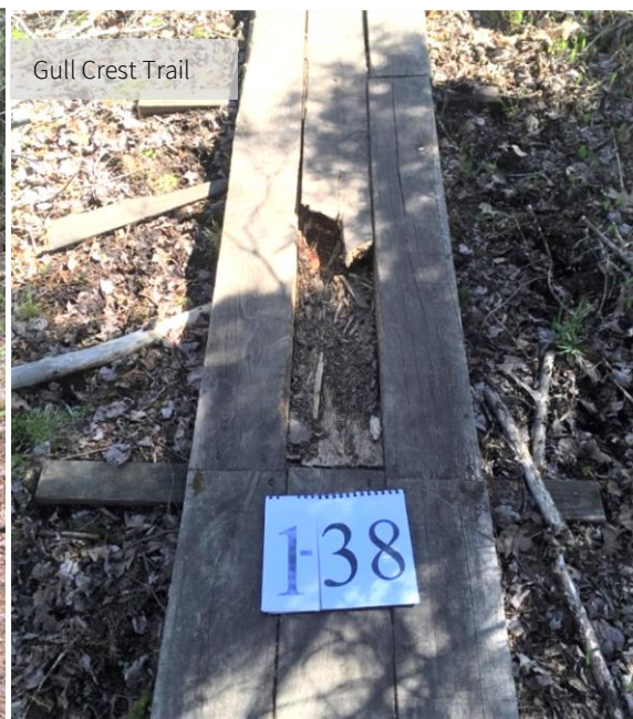
Photo 10. Example of high priority repairs. Site 1-38 requires more than ten repairs similar to this.
