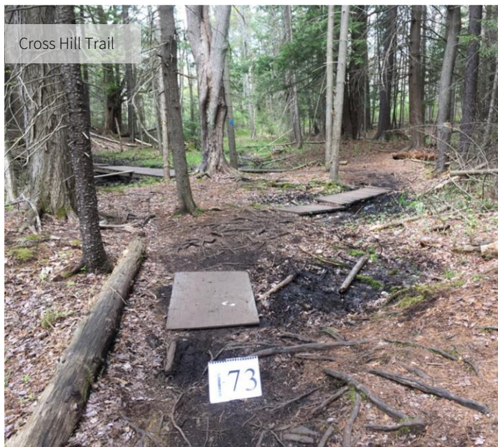
Photo 9. Example of high priority boardwalks lacking foundations.
