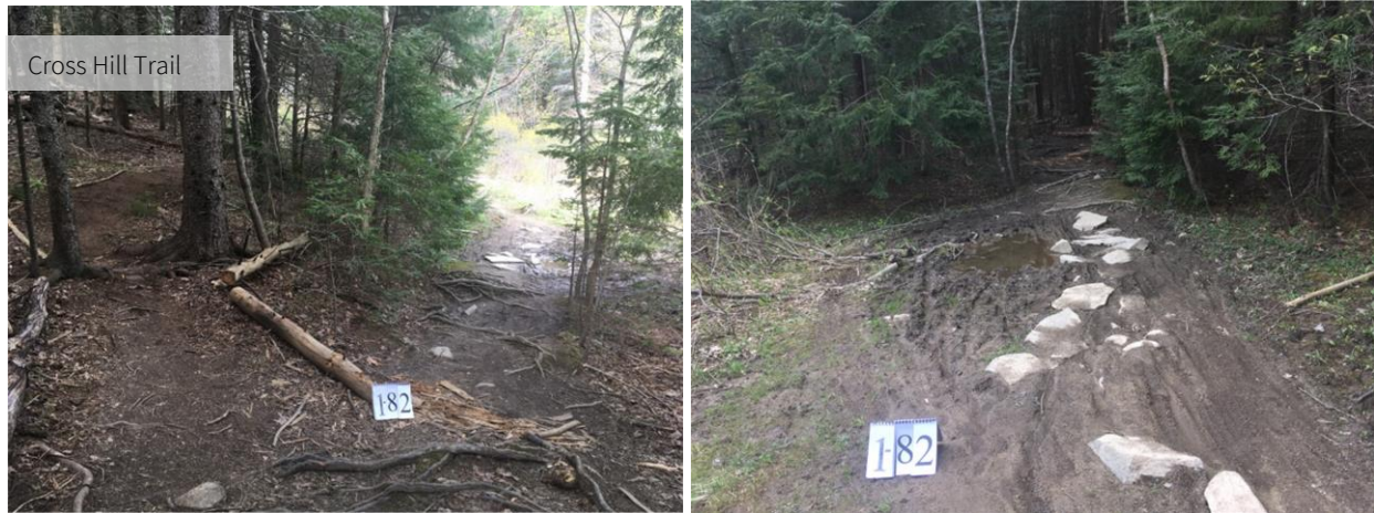
Photo 4. Example of a trail assessment site viewed from above (top) and below (bottom) with a recommendation to re-route the trail or install a new boardwalk. In this example, the re-route appears to already be partially established by trail users and could be fully established with confirmation of land access rights.
