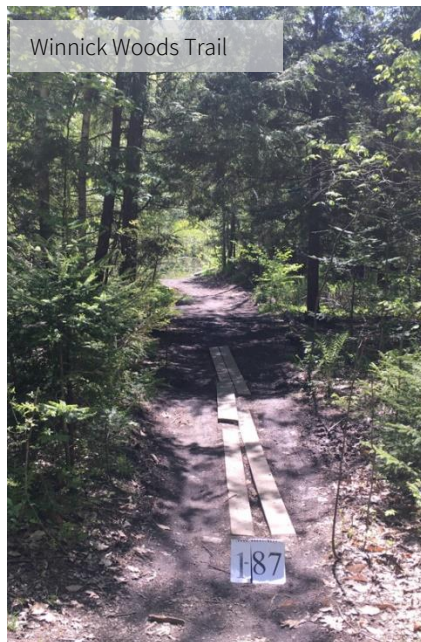
Photo 1. Boardwalk site with no proper foundation, rated at a 4 on the boardwalk condition scale due to loss of some function.
