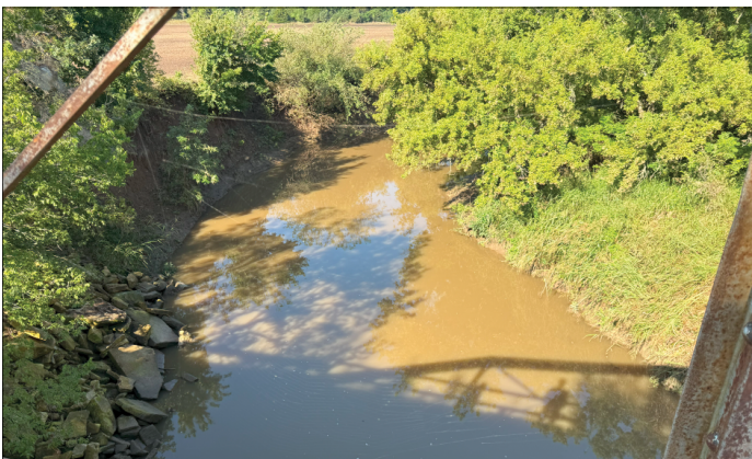
(2) Channel looking West (see embankment scour and existing riprap)
